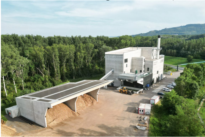
Biomass-fired cogeneration plant
